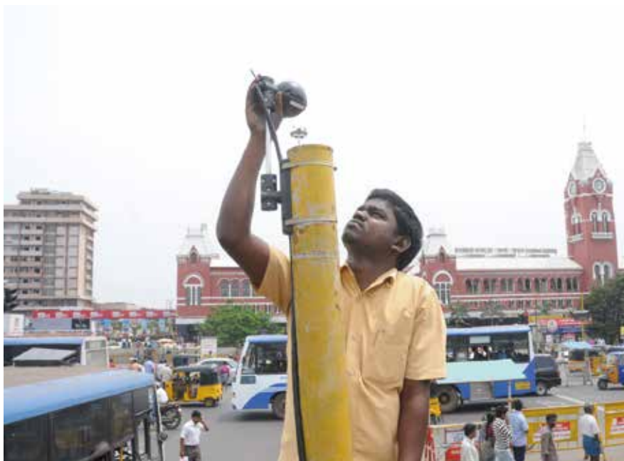
Installation of a FLIR TrafiCam sensor.
