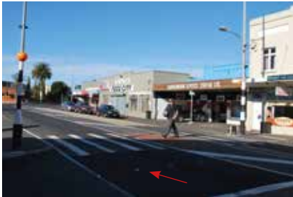
FLIR's C-Walk and SafeWalk video sensors activate on-road markers along a zebra crossing when a pedestrian is in range.
