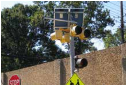
FLIR C-Walk installed at the top of the traffic lights.
