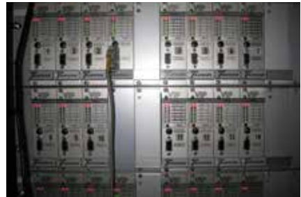
A rack with integrated VIP cards.
