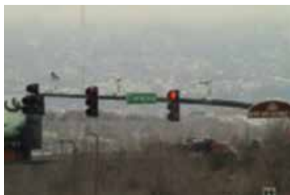
FLIR VIP-T modules are used for vehicle presence detection & traffic data collection in Colorado Springs.
