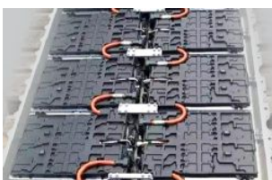
Battery charge/discharge test
